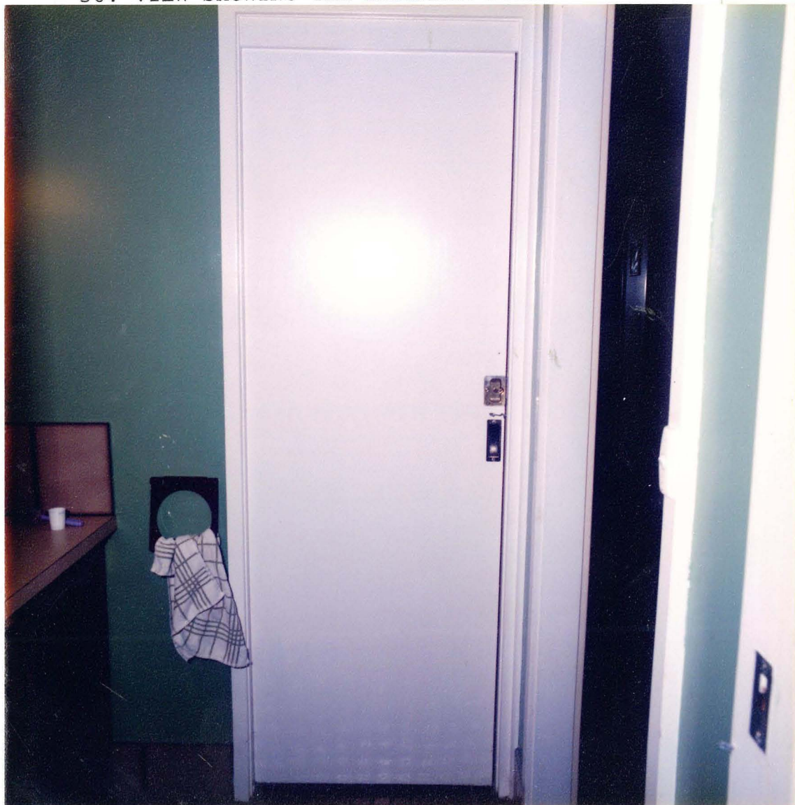
36. VIEW SHOWING THE BATHROOM DOOR.
